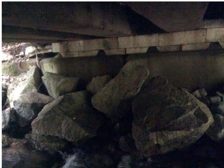
Left Bank Abutment when facing downstream
