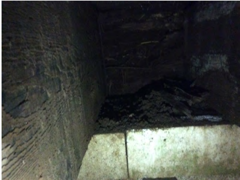
Left Bank Abutment when facing downstream
