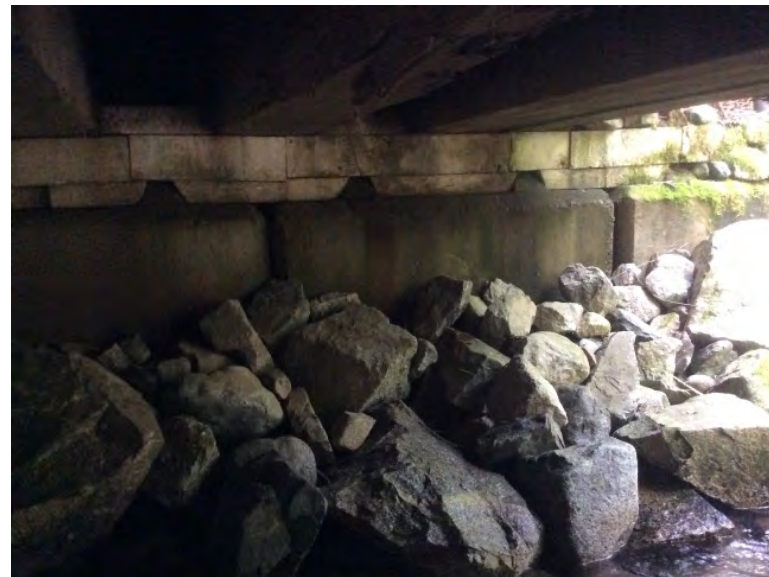
Right Bank Abutment when facing downstream
